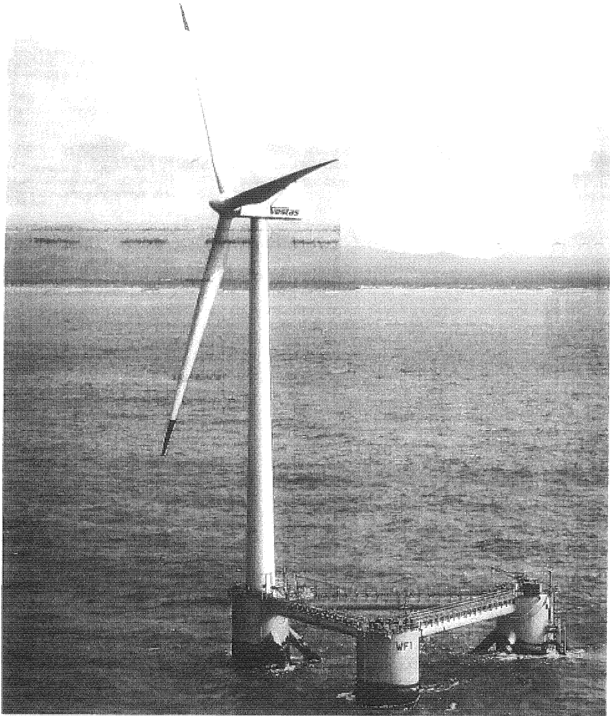
Wind instruments: semi-submersible platforms have been trialled off Norway and Portugal - © Kate Pridmore / Getty Images
